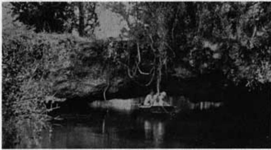
The County Road crossed Arch Creek on the famous natural bridge. Photo about 1900. — Photo in collection of HASF Museum
