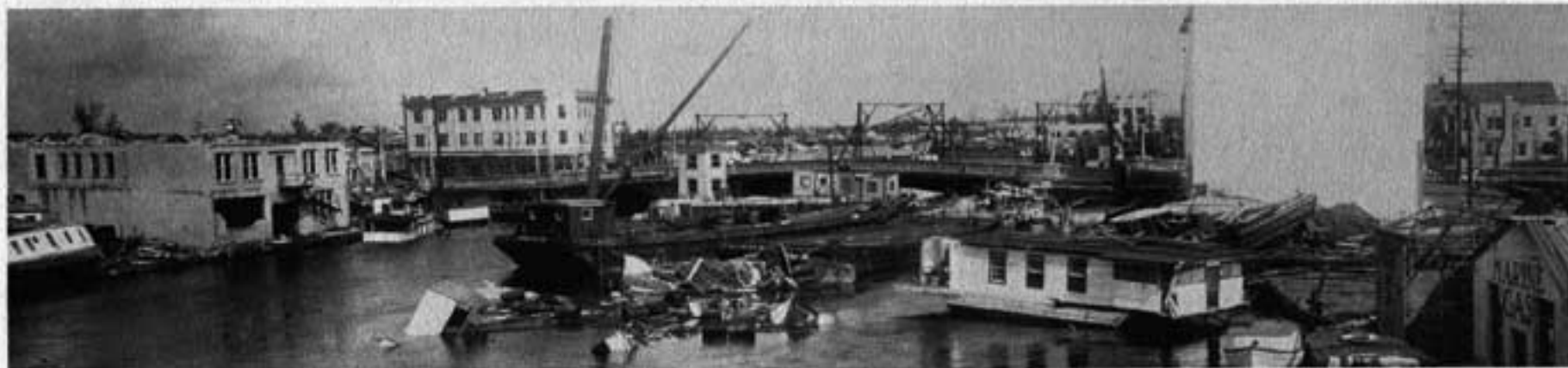
The Miami River at the Flagler Street Bridge was left a mass of tangled debris after the 1926 Hurricane. The building in the far right hand corner is the Scottish Rite Temple on N.W. 3rd Street. —Photo collection of HASF Museum
