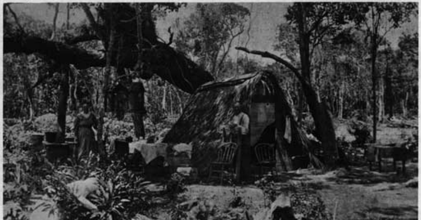
This palm-thatched A-frame with mosquito netting door and outdoor cookstove and pantry was typical of the housing for hundreds of workers who came to Miami during the first boom. In 1896 the population went from near zero to 2,000. — HASF Museum collection.
