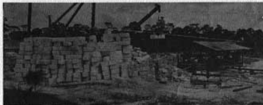
The Offer-Cronkhite Quarry Company, located near the present S.W. 8th St. and the railroad, supplied oolitic limestone blocks for the 1904 courthouse.
