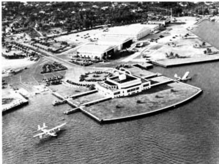
By 1934 Pan Am had built two hangars now leased by Grove Key Marina and Merrill Stevens and the terminal building which is now Miami's City Hall.
