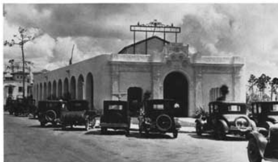
Coral Gables Post Office, another DeGarmo building in 1926.
