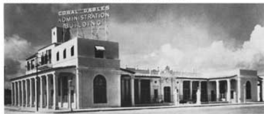
Coral Gables Administration Building, built by DeGarmo, was photographed in 1925 from NE Coral Way.
