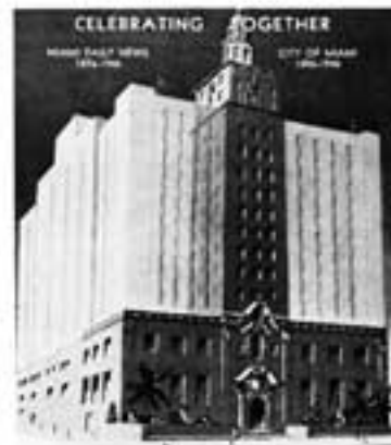
In 1946 50th anniversary program The Miami News published sketch of proposed expansion of News Tower similar to recent hotel plans. (NASF)
