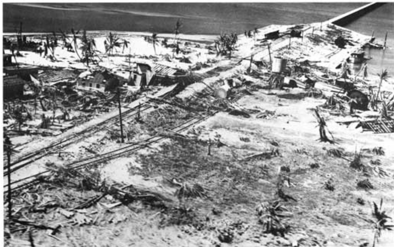
Lower end of Long Key and Long Key viaduct. High water floated railroad ties which were caught by the wind, overturning the rails. (MASF, gift of Mrs. Karl Voelter)
