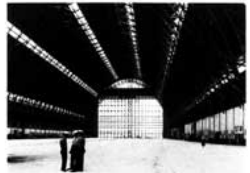
1945. Richmond Naval Air Station had three huge blimp hangars, made of wood except for concrete and steel doors. In the storm they broke up and caught fire. Destroyed were 25 blimps, 366 aircraft and 150 automobiles. (NASE, courtesy of the Miami News, negative number 81-99-41)
