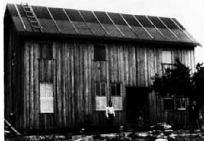
The Richmond Hotel, still under construction in this picture, was remodeled to contain the kitchen and dining room for the Deerings after the buildings were joined. (HASC gift of Kay Pancaost, negative number 74-8-1)
