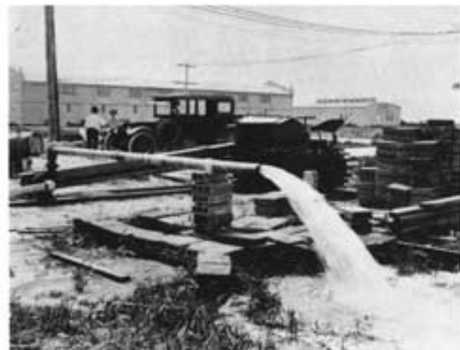
Test of drinking water wells in Miami Springs.
