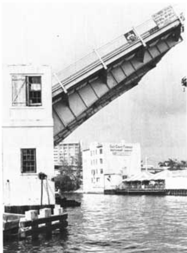
First Street Bridge with East Coast Fisheries in background.
