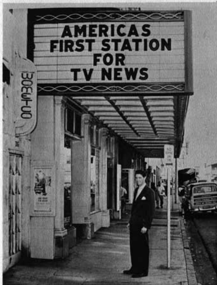
In 1952, the famous Capitol Theatre was converted into a TV station - WTVJ. The largest studio in the South and one of the most complete in the nation at that time, Studio A was built within the framework of the old theatre, which was next door to the original station. Here a younger Ralph Renick poses in front of the building.
