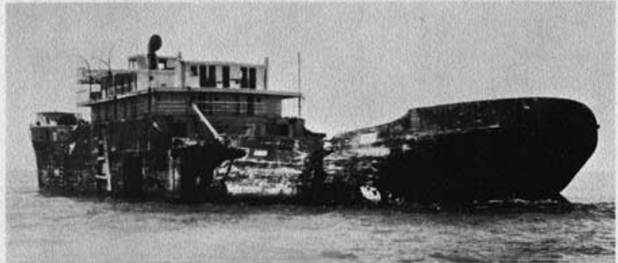
An old concrete ship aground near South Bimini became a convenient liquor warehouse for rumboats. (Photo from the HASF Collection).
