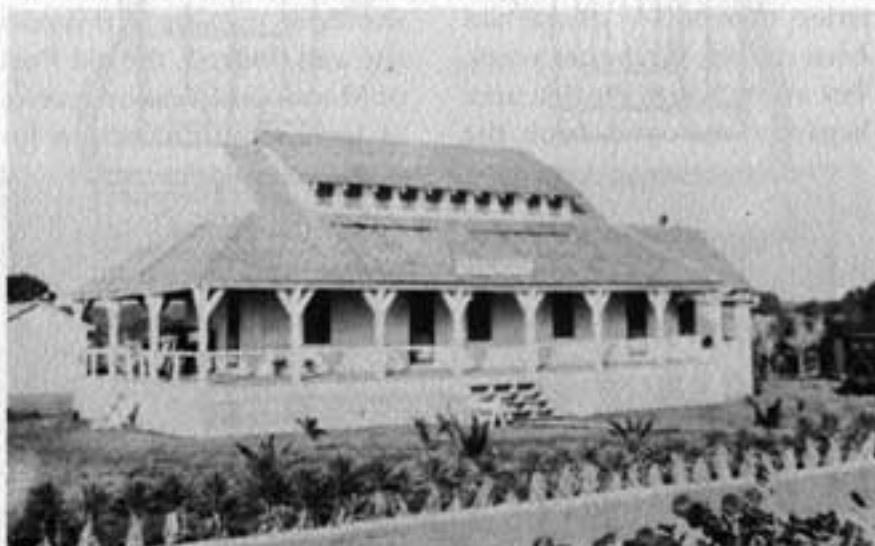
The first floor of the Biscayne House of Refuge was living quarters for the keeper and his family. The second floor loft was to house stranded seafarers.
