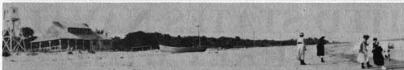
The Biscayne House of Refuge was built in the area known today as Surfside. The keeper was responsible for patrolling the coast from Norris Cut north halfway to Ft. Lauderdale after storms. This photo was taken in 1918. Eight years later the refuge was destroyed in a hurricane and was not rebuilt.
