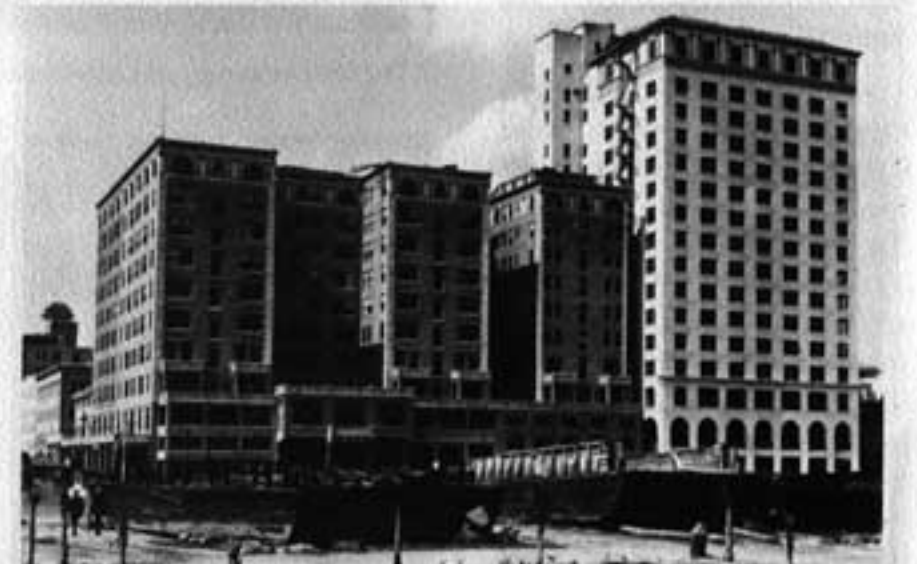
Three barges were washed ashore on Bayshore Drive (Biscayne Boulevard today) in front of the McAllister and Columbus Hotels.
