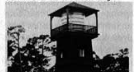
The windmill tower at the rear of Munroe's Grove home served as his studio. The room at the top of his "Tower of London" was where Munroe wrote his books and entertained neighborhood youngsters with stories of his adventures. (Photo courtesy of Arva Moore Parks.)
