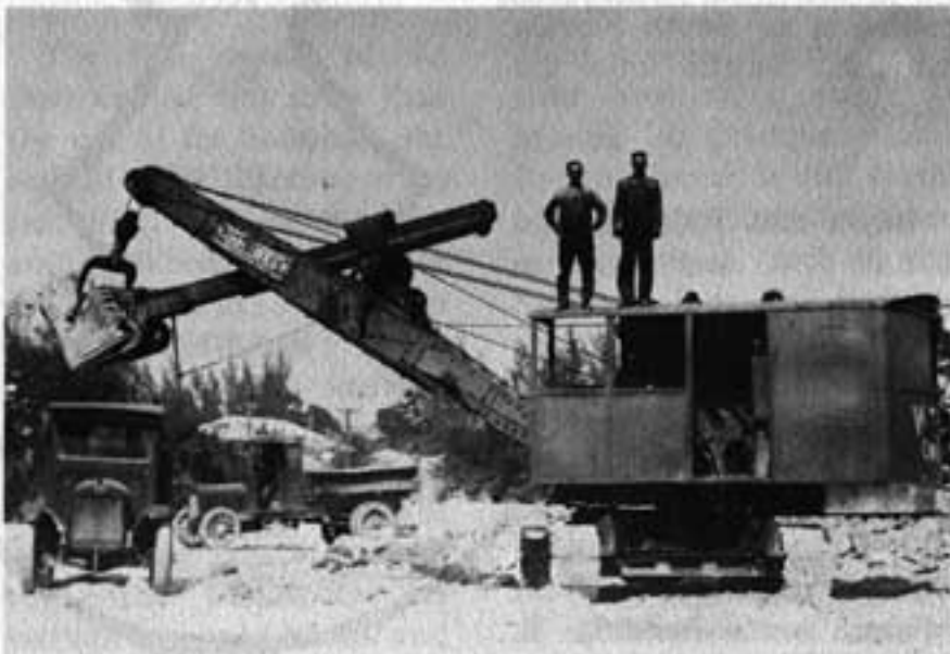
William G. Castleberry and H. E. Crawford took time out from building McFarlane Road on October 23, 1925 to pose for the Illustrated Daily Tab . (All photos courtesy of the Romer Collection, Miami-Dade Public Library.)
