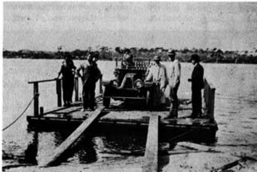
The Highleyman family crosses an inlet on their way to Miami. After driving their car onto the barge, called a cable ferry, they were pulled across to the other side. (Photo from the Highleyman Collection; Katherine Highleyman, photographer.)
