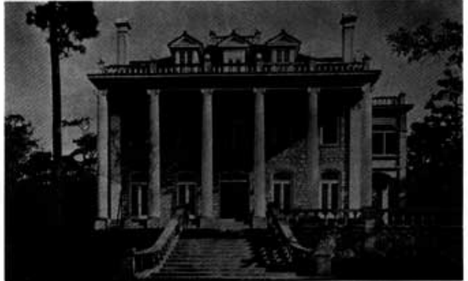
Construction on Hallssee Hall began in 1912. The "Miami stone" used in building the house came from the property, the highest point of land in the city. Walls of the home were 18 inches thick and Hallssee Hall's third floor was a ballroom. Today the landmark is part of the Jackson Hospital Medical Complex. (Photo from the HASF Collection.)
