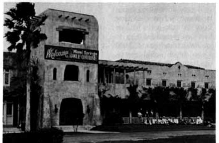
The Miami Springs Golf Course Club House was a good example of that city's "pueblo" architecture theme.
