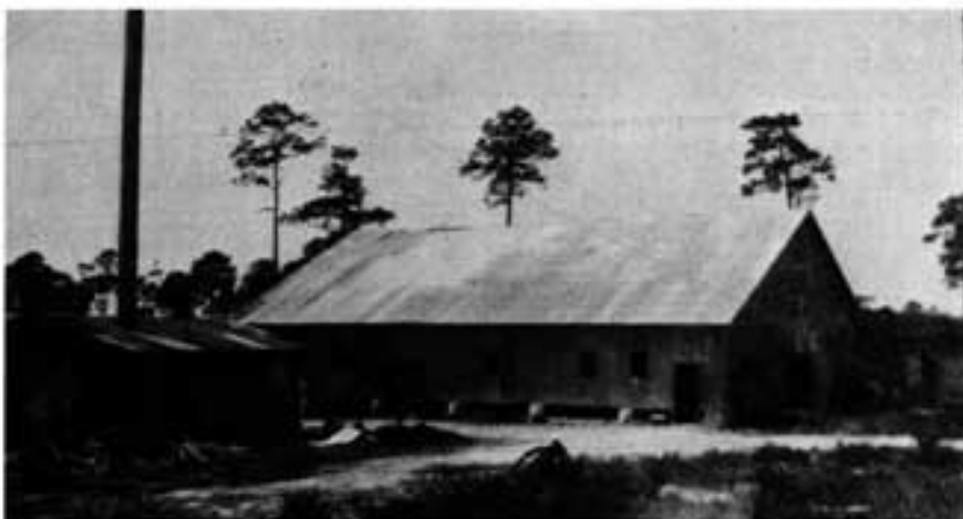
The factory and boiler shed of the A. B. Hurst Co. produced "Florida Arrowroot Starch." The powder was used by soldiers in W.W. I and later was considered a good nutrition source for children.
