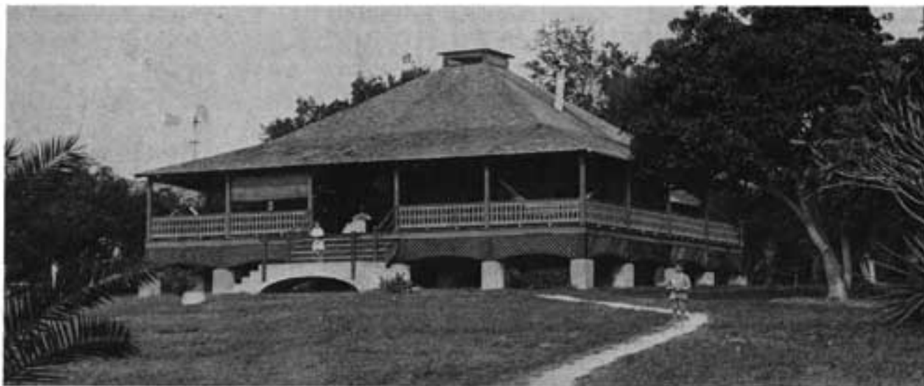
Jessie Munroe is joined by her children in front of the Barnacle. In 1908, the Commodore raised the bungalow and built a cement block first floor underneath. The family lived in Banyan Cottage at Camp Biscayne while the work was progressing. Photo © Munroe Collection, 1977.
