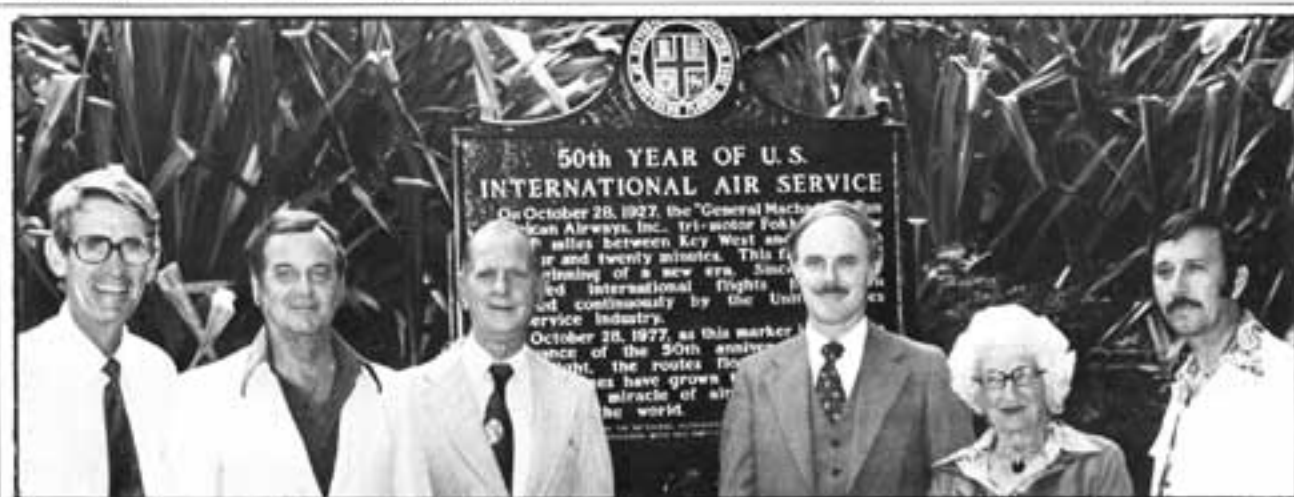
The historical marker commemorating fifty years of international air service was dedicated on October 28, 1977, in Key West. Gathered in the patio of the Historical Museum, East Martello Tower for the dedication were (left to right) Charles Munder, Key West Art and Historical Society; Charles McCoy, Mayor of Key West; Joe Allen, State Representative; R. Layton Mank, President of the Historical Association of Southern Florida; Ione S. Wright, HASF Board Member; and Wright Langley, Historic Key West Preservation Board. (See story on page 9). (Photo courtesy of Pan American Airways.)
