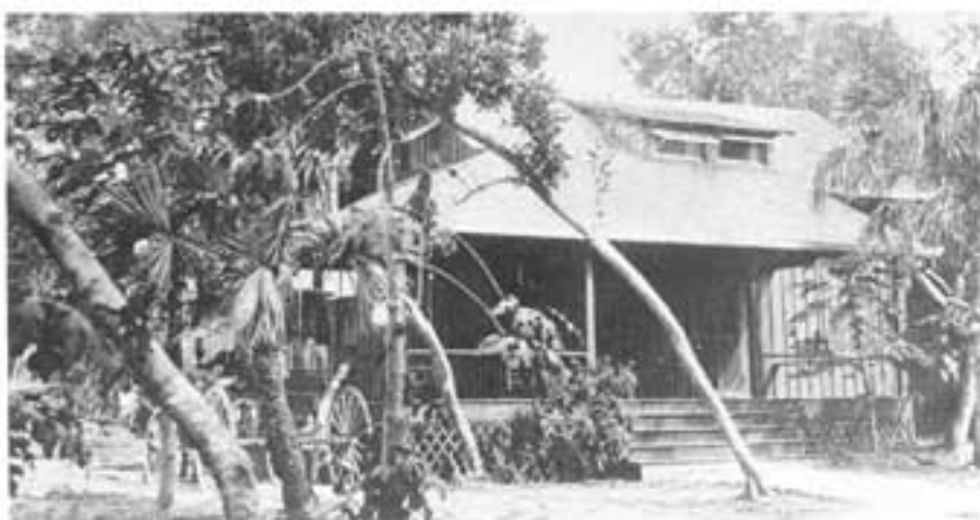
Orchid Cottage at Camp Biscayne was advertised as "a large, rambling cottage with four rooms and bath on the lower floor and three rooms on the second floor. Especially adapted for a large family." The original main dining room and kitchen for the Camp were located in the cottage. (Photo courtesy of Patty Munroe Catlow.)
