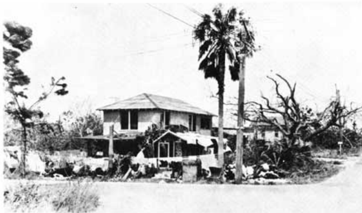
"L. Tillotson after the hurricane. Sept. 18, 1926 at Coconut Grove, Fla. Clothes, bedding, etc., drying. Yard is piled with limbs from the large pithecolobium tree. Washingtonian Palm broken off and laying against roof of porch which it broke. Pine tree broken off in front yard. No leaves on fruit trees. Roofing paper gone. House soaked. Window lights out, awnings damaged, copper screens gone. Center of large porch roof sags. Virginia and Day Ave. N.W. Corner." Editor's Note: The Tillotson home was located at 3009 Day Avenue. (Photo HSAF Collection. Courtesy of the City of Miami Fire Department)
