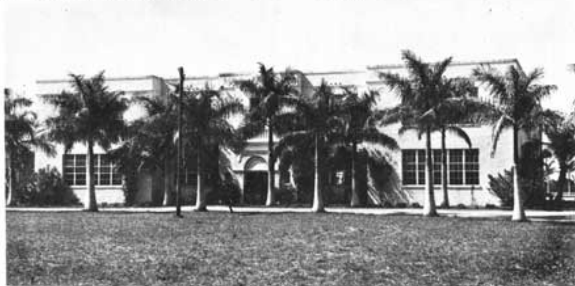
The two-story Spanish style Redland High School was built in 1927 to handle the expanding student population. The school became a junior high facility in 1953 and is presently being enlarged and remodeled.
