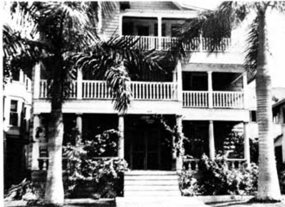
Additions to the building included a third floor veranda on the front and a tier of screened porches on the east side.
