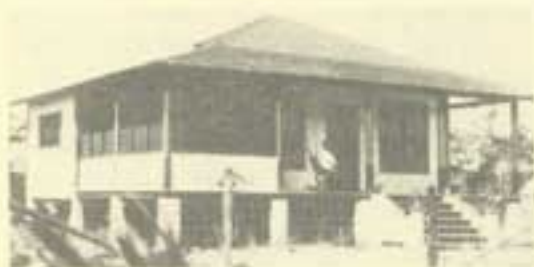
Basic Cracker: Greenwood house in the Grove is off the ground, has high-pitched wooden roof, porch.
