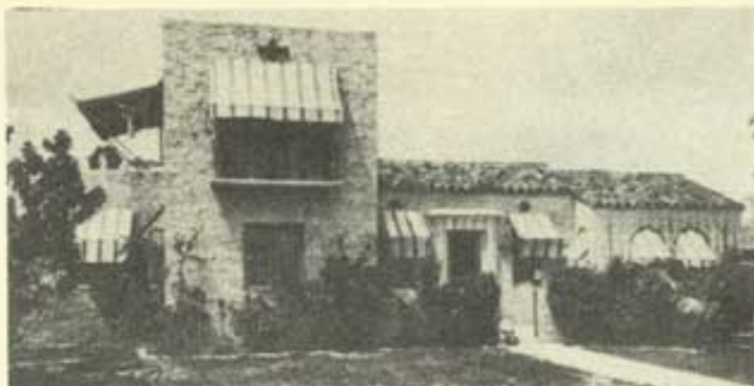
Spanish: no overhangs; homeowners added awnings that darkened house, required replacements.
