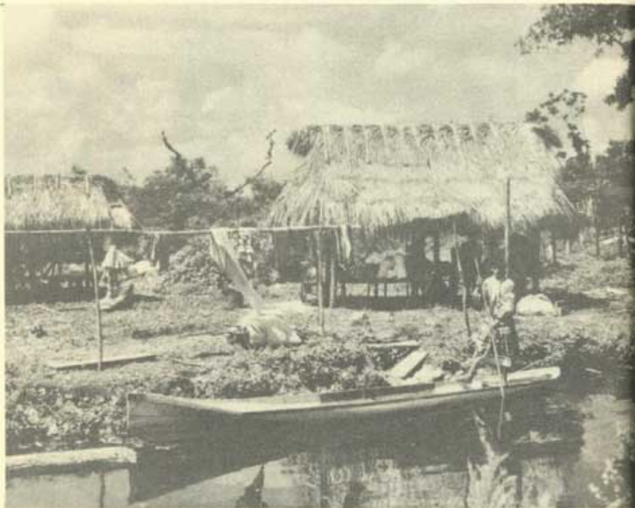
Chickee made of native palmetto fronds and Dade County pine has overhang against sun and rain and plenty of cross ventilation.
