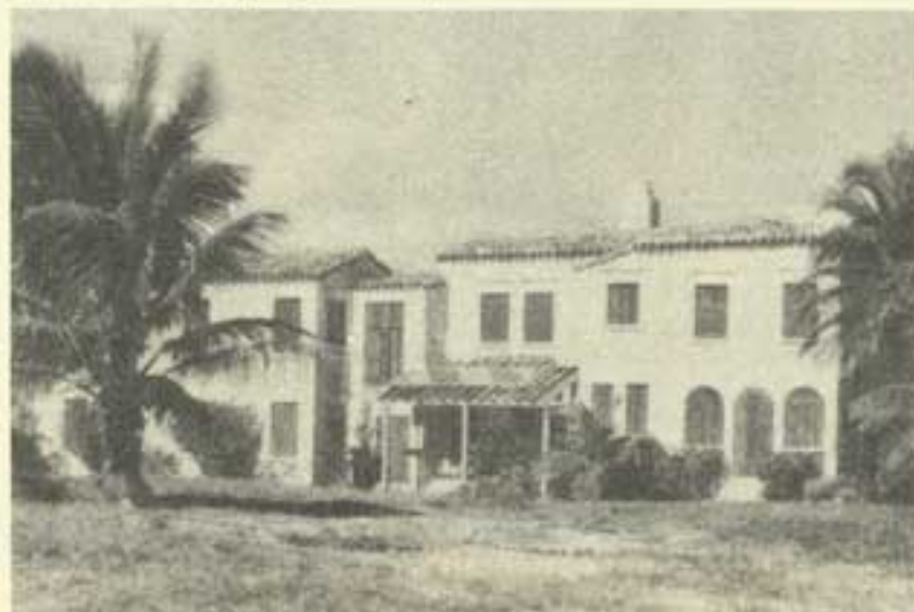
Solar Heat: device for heating water is installed on shed roof of this 1920s home.
