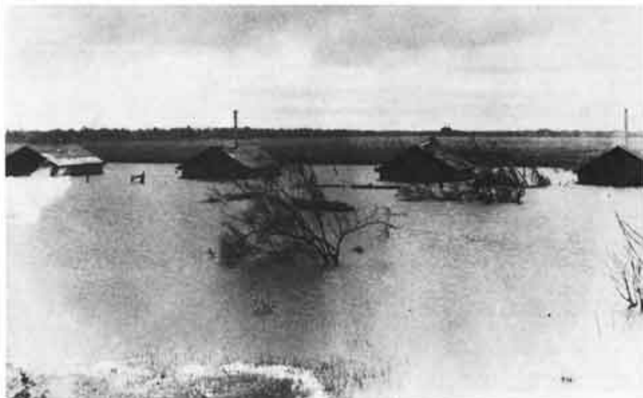
Two wet hurricanes in 1947 left 15,000 square miles of South Florida flooded. Suburbs of expanding cities were set out in the old basin of the Everglades. Farms and groves were drowned; cattle starved. This is Cooper's Chicken farm north of New River canal, September 1947.
