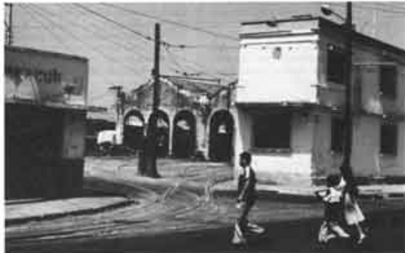
High-arched openings are facade of the trolley barn of the Sociedad Cooperativa, set behind buildings that line a commercial street in Veracruz, Mexico.
