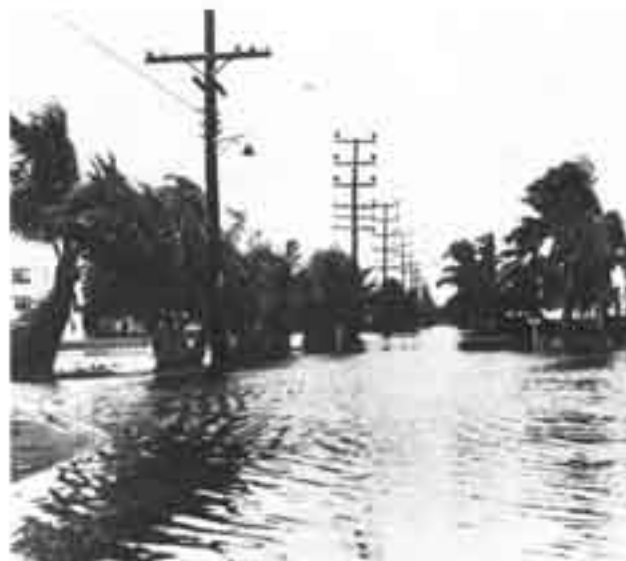
Harding Ave. intersection on Miami Beach became a lake.
