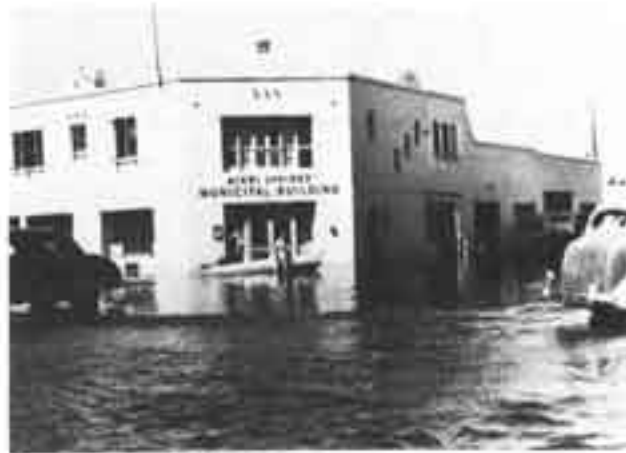
Canal overflowed in Miami Springs. Winds reached 80 mph at airport.
