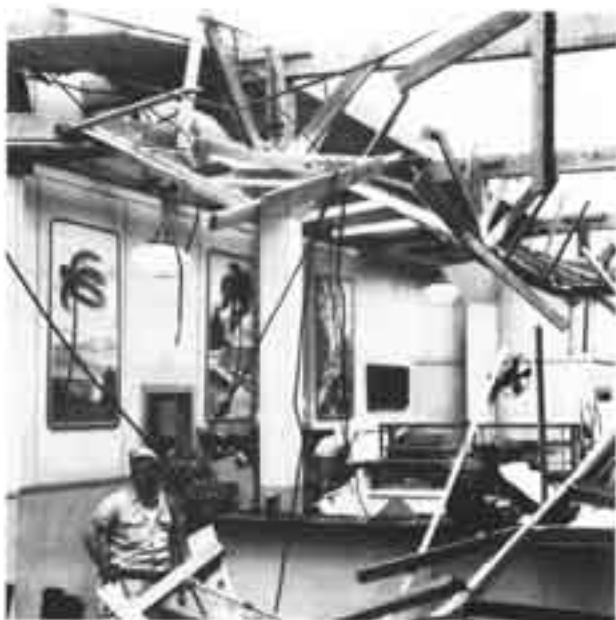
Homestead AFB shows effect of 104 mph wind in 1945's third hurricane.
