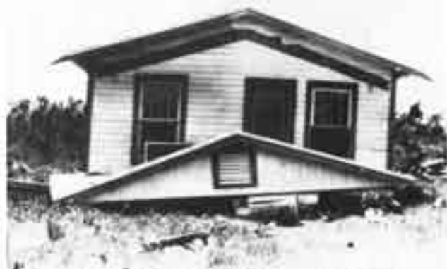
Hathaway House. John Talbott wheeled the mail to the train every day in a wheelbarrow.
