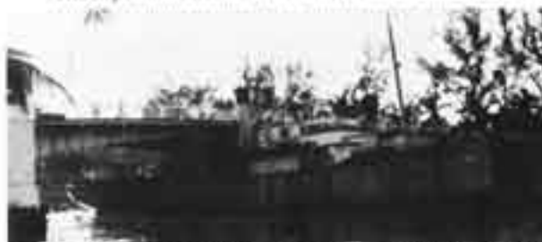
SE 2 Ave. bridge damaged by banana boat in second 1948 storm.
