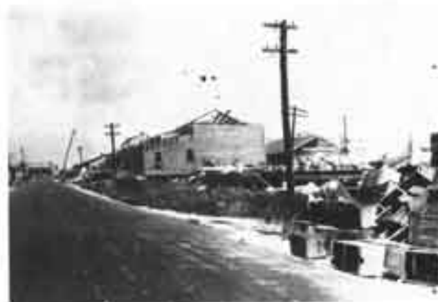
Burr and Bush packing house was among devastation in Goulds after storm.
