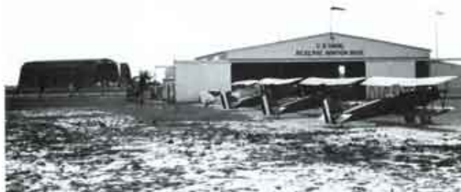
Opa-locka, one of four local Naval air bases, had a blimp hangar in 1931 photo.
