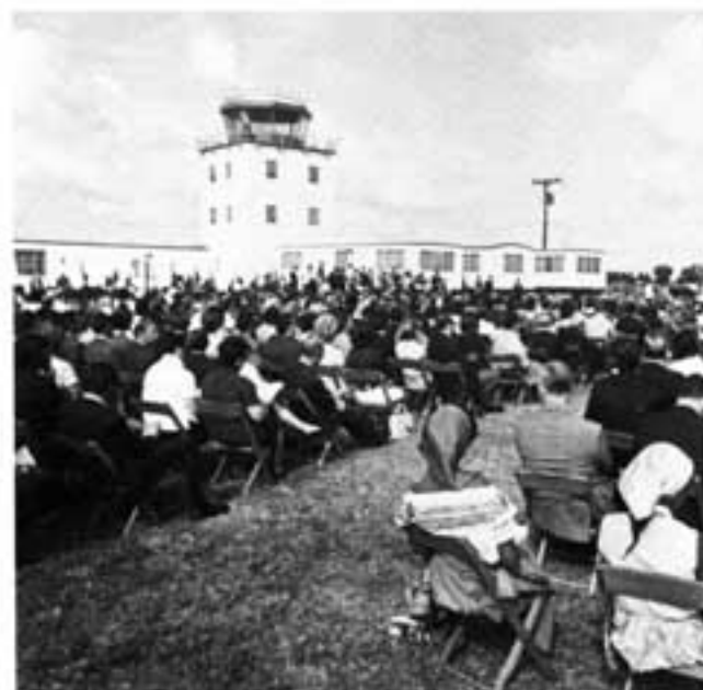
Perry's Ivory Tower - The control tower which the planning team took over surrounded by a cluster of mobile units.
